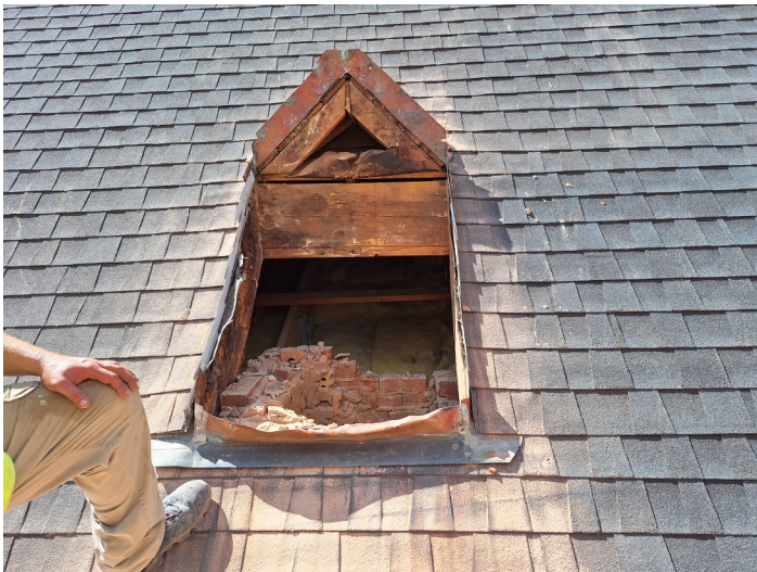
Chimney demo continued
