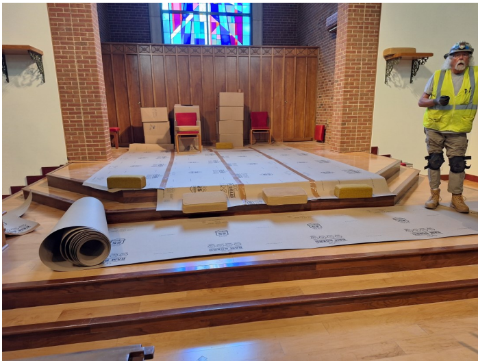
Altar protection in progress
