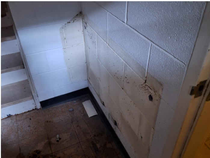
FCU removed in back hallway by the Alter
