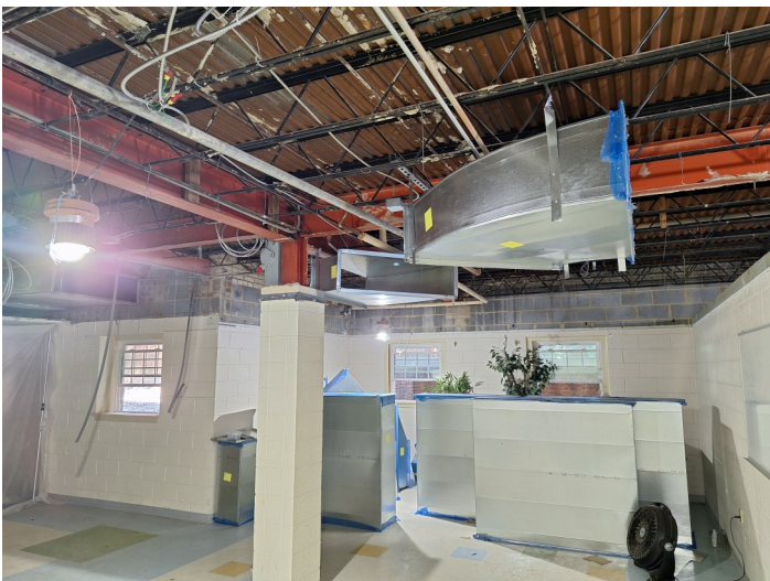
Ductwork installation
