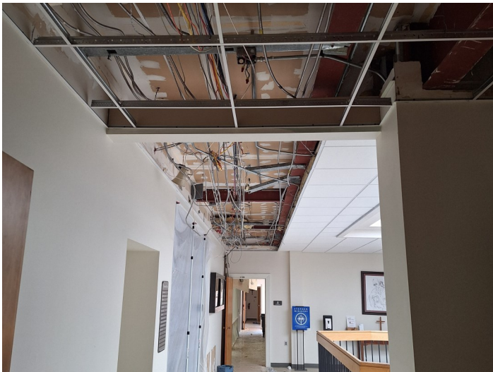
Ceiling removed in the choir corridor
