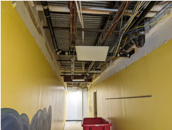
Corridor grid and tile removed
