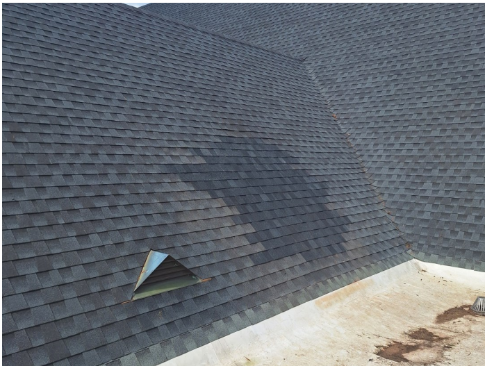
Chimney penetration repaired
